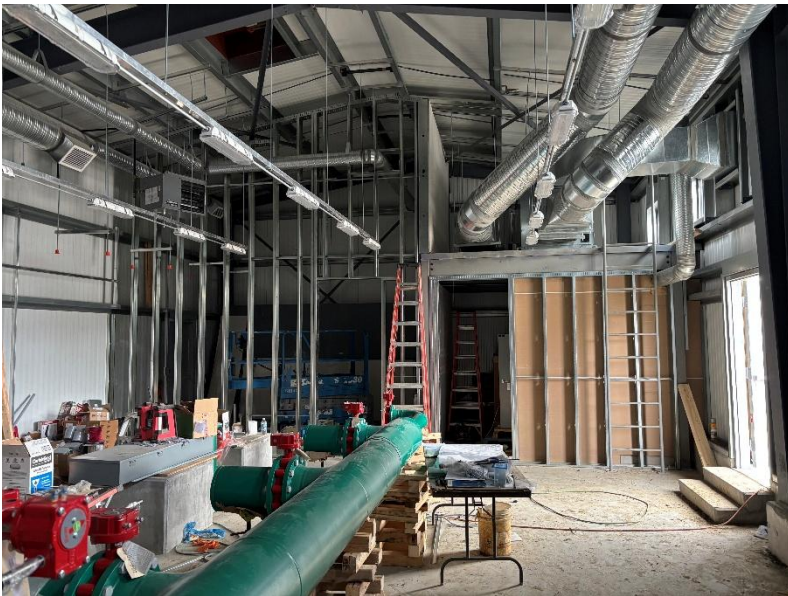
June 11 th , 2026. Ongoing Process Piping.
