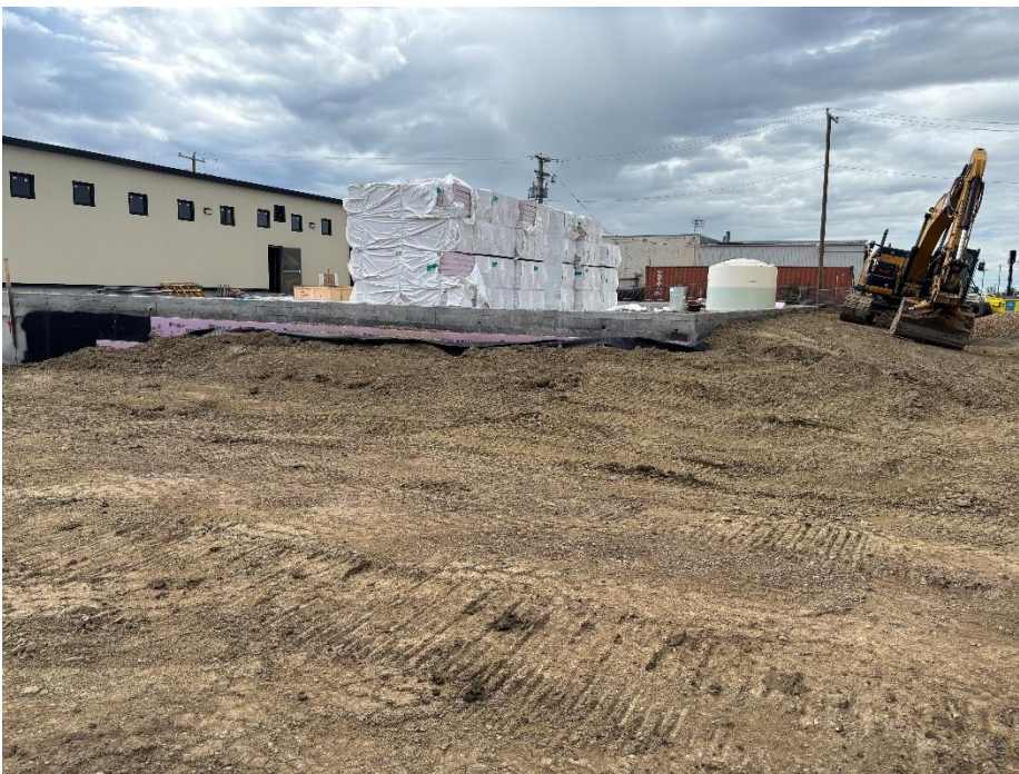
June 11 th , 2026. Continued Backfill Operations.
