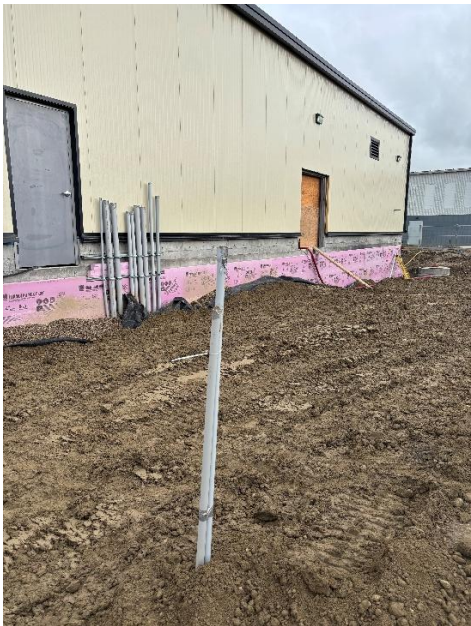
June 11 th , 2026. Backfill.
