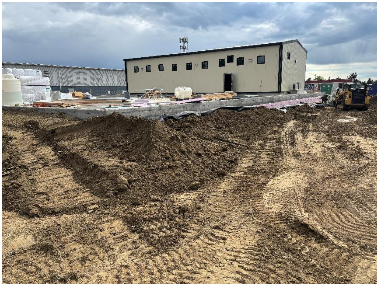
June 11 th , 2026. Backfill.
