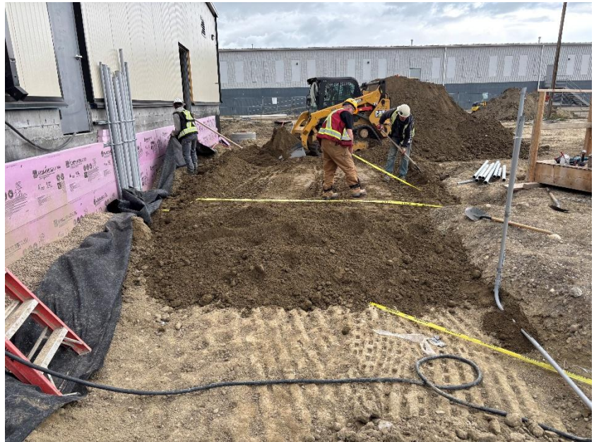
June 11 th , 2026. Backfill Operations
